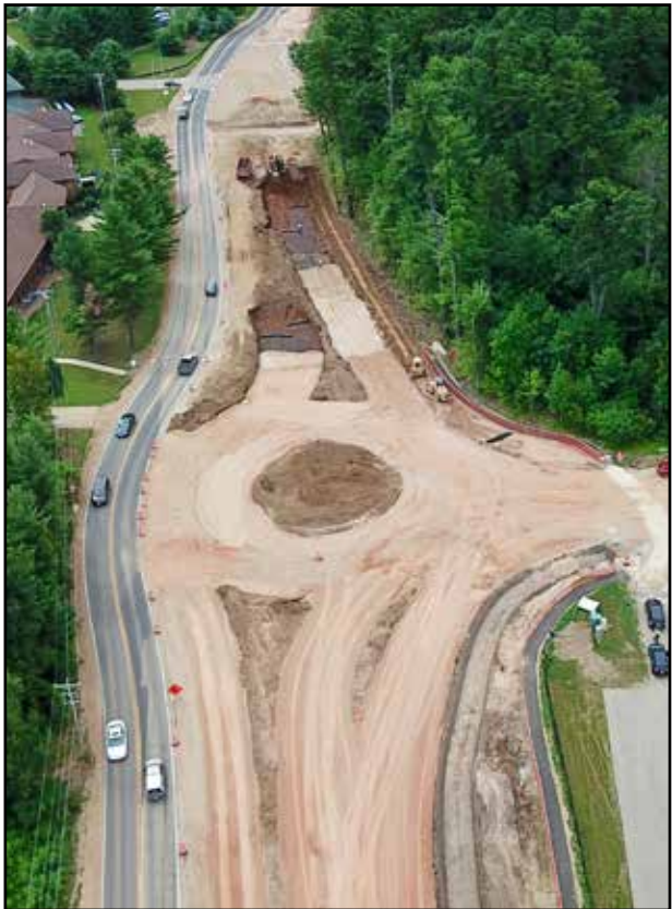
The Wisconsin Department of Transportation (WisDOT) worked in cooperation with the Menominee Nation to construct a roundabout on Highway 55 in Keshena, Wisc, which created a safer and more efficient way to enter the Menominee Casino Resort. (Photo courtesy of WisDOT.)
